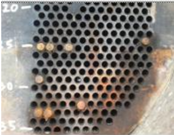
Gambar 4. Plugging tubes condenser (sumber ; PT PJB UP Gresik, 2014)
