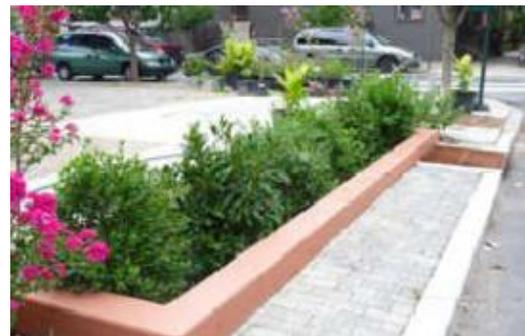
Gambar 8. Contoh stormwater planter di Columbus Square, Philadelphia, PA.
