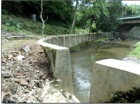
**Gambar.3** Tembok Penahan Tanah (*Retaining Wall*) Restorasi Sungai Cikapundung
