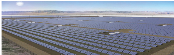
Gambar 18. Sistem Grid-connected centralized
