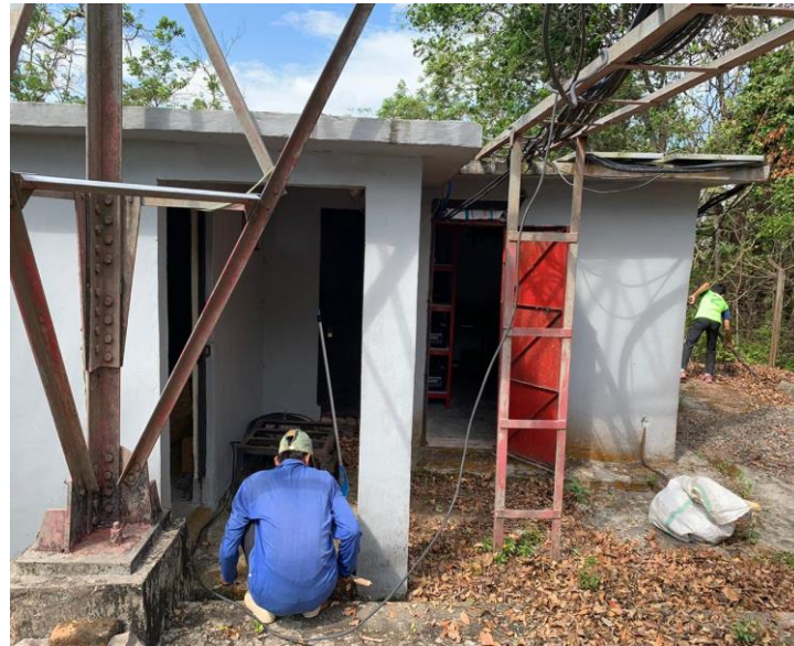
Gambar 3. Shelter Radio Repeater Mattirowalie Tampak Depan
